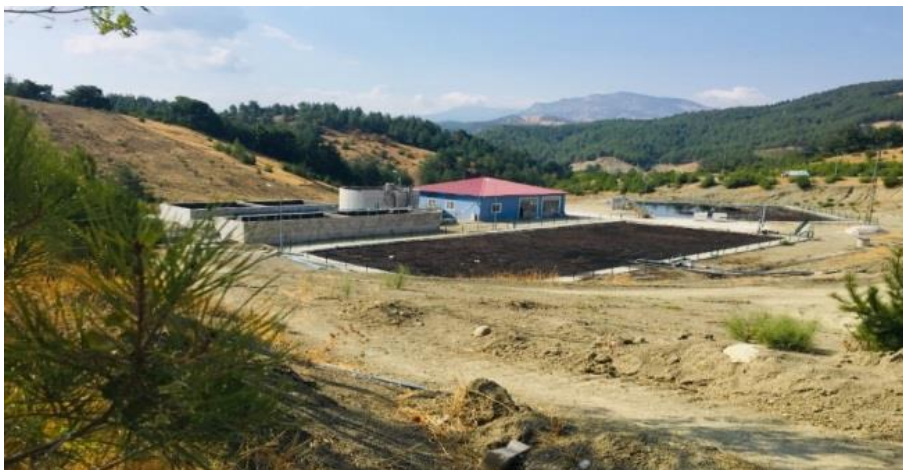
Fig. 2. Treatment plant overview.
