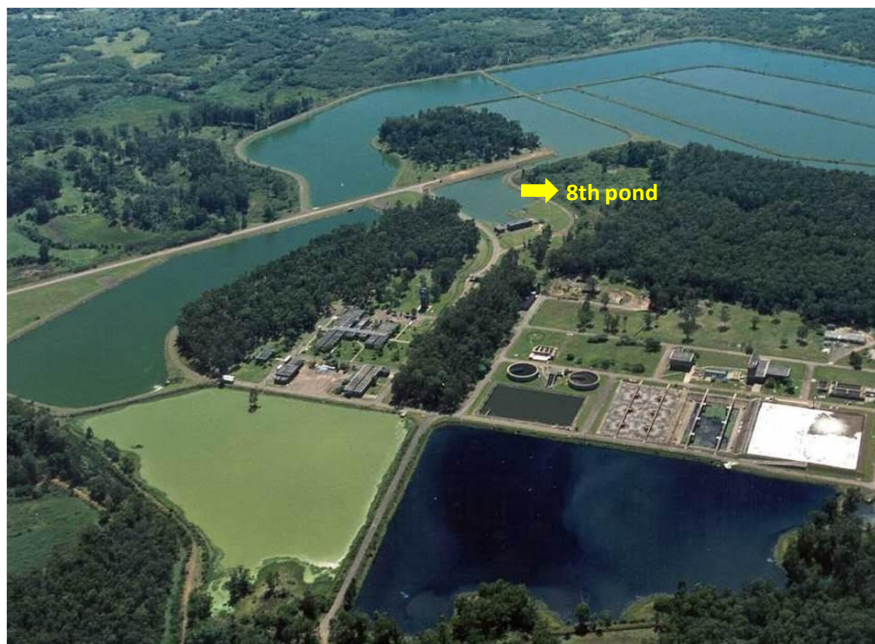
Fig. 1. Aerial view of the wastewater treatment plant showing the collection point.
